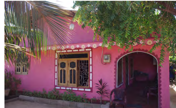
Permanent housing located in the central area
