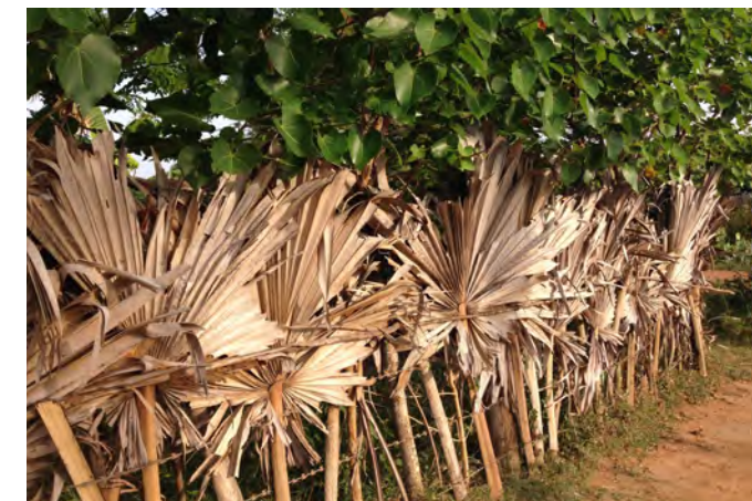
Temporary fencing made from Palmyra, a local product
