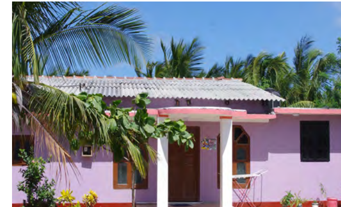
Permanent housing located in the central area
