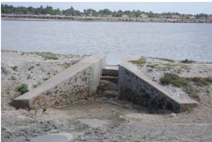
Box culvert to salterns
