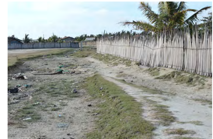
Encroachment of fence property into the drainage
