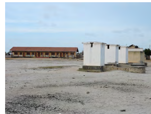
School grounds can be raised; this will allow people to access the bathrooms during the rainy season
