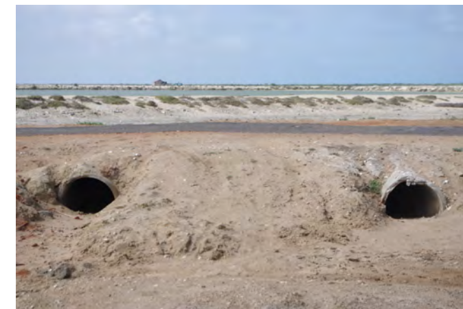
Block drainage under Station Road
