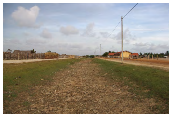
Old Dutch Canal running north south (northern section)
