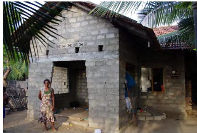
Permanent housing located in the central area
